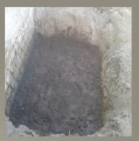
2. - Poor concrete pavers. A lean concrete f'c= 150 kg/cm2, will be placed, to avoid contaminating the concrete of the footing.
