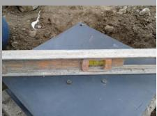
7. - The slab is placed on the upper part of the insulator.Carefully join the insulator and the slab with a 3/8" smooth rod.
