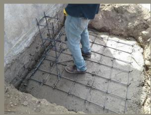
4. - Concrete f'c= 250 kg/cm2 will be placed over the entire footing; taking care that the upper part is level.
