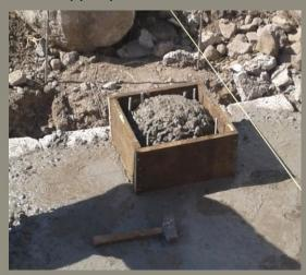
5. - Grout placement. A grout layer will be added so that the steel plate is completely level.
