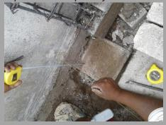
6. – Insulator placement. Once the grout is poured and checked everything is level, the seismic isolator is placed.
